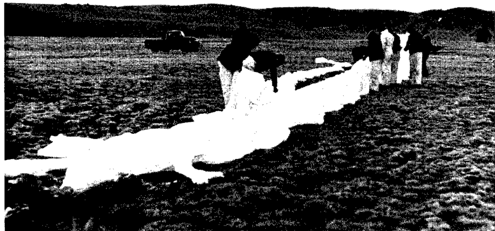
Fig. 79. “Stretching stuff out on the ground, dragging stuff out of trucks”—a likely witness reference to high altitude balloon inflation procedure that required the balloon to be stretched out on a protective ground cloth prior to inflation. (U.S. Air Force photo)
